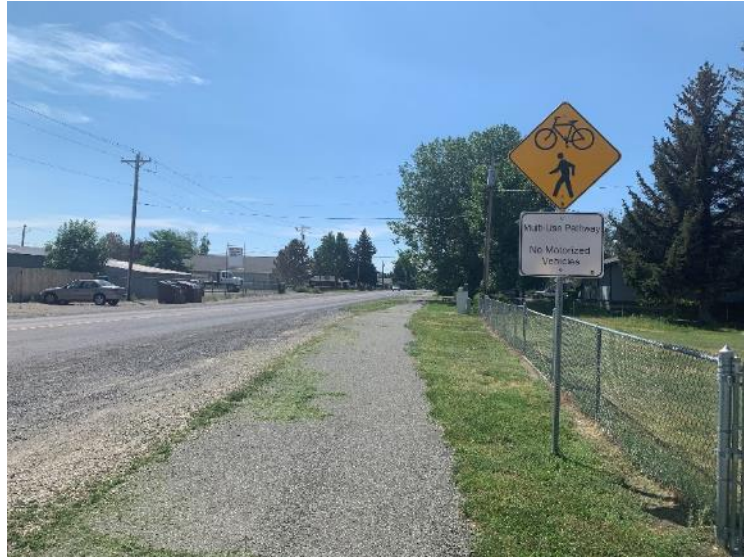
Figure 36. Paved pathway along 29th Street
