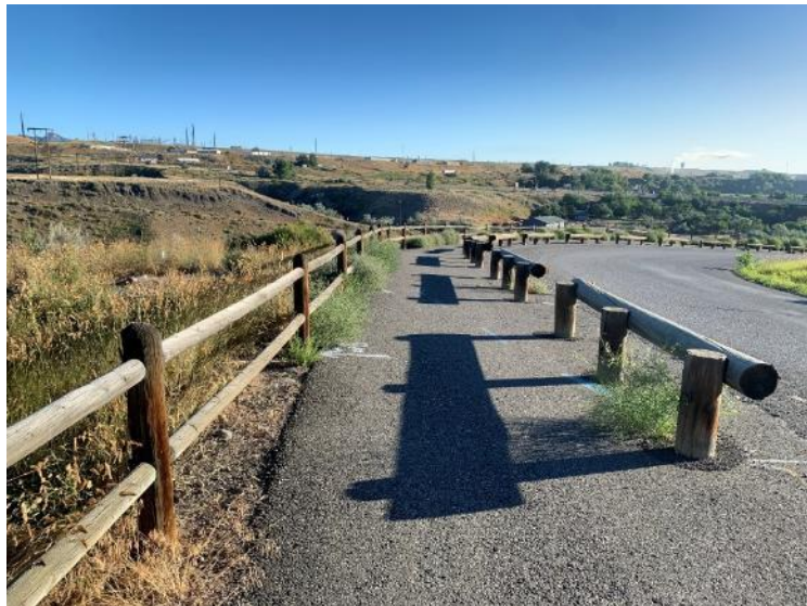
Figure 37. Paved pathway with vertical separation along 12th Street
