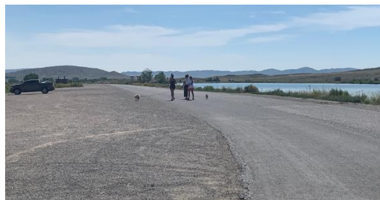
Figure 38. Paved pathway at Beck Lake Park
